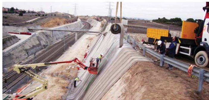
Figure 1. Concrete Canvas used for slope lining
